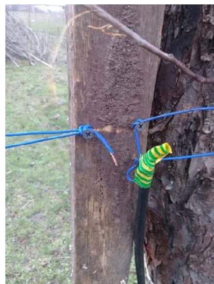
Figure 5 Feeding of the Simple Vertical Antenna
